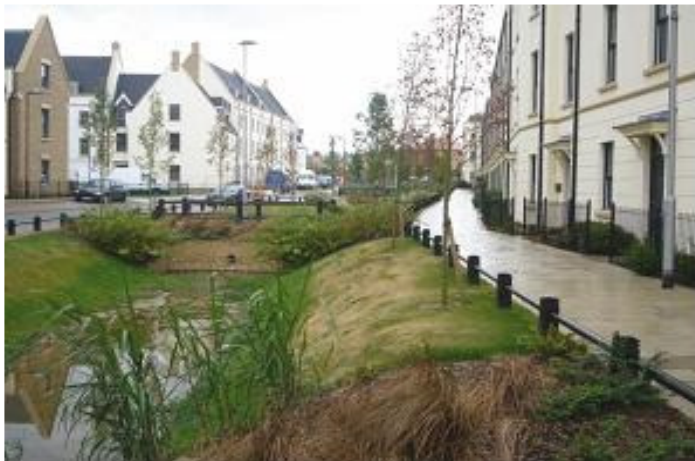
Water cycle management integrated with the built environment at Upton urban extension,
