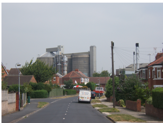
View of former British Sugar site from Plantation Drive
