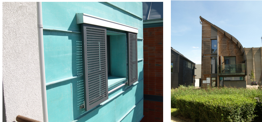
Sustainable housing at the BRE centre.
